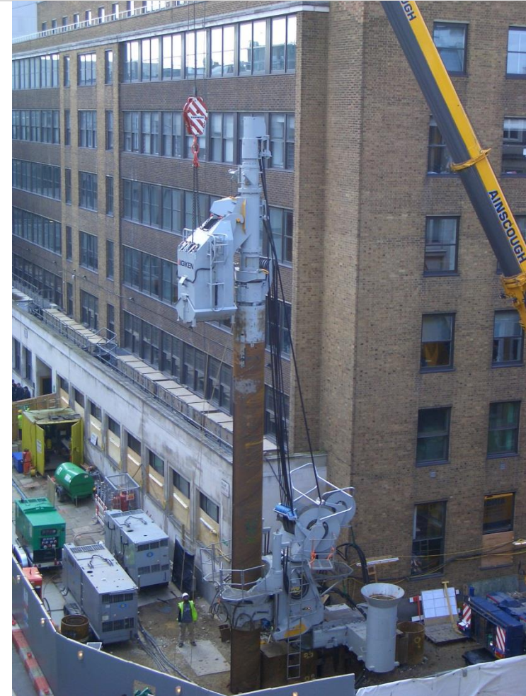
BBC, Central London Sheet Piling Works in Commercial Area
