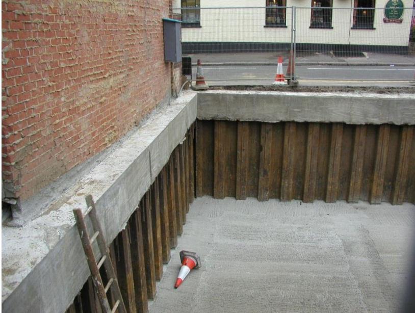
Steel Sheet Pile Wall
