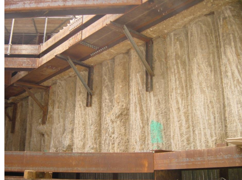
In-situ Concrete Pile Wall
